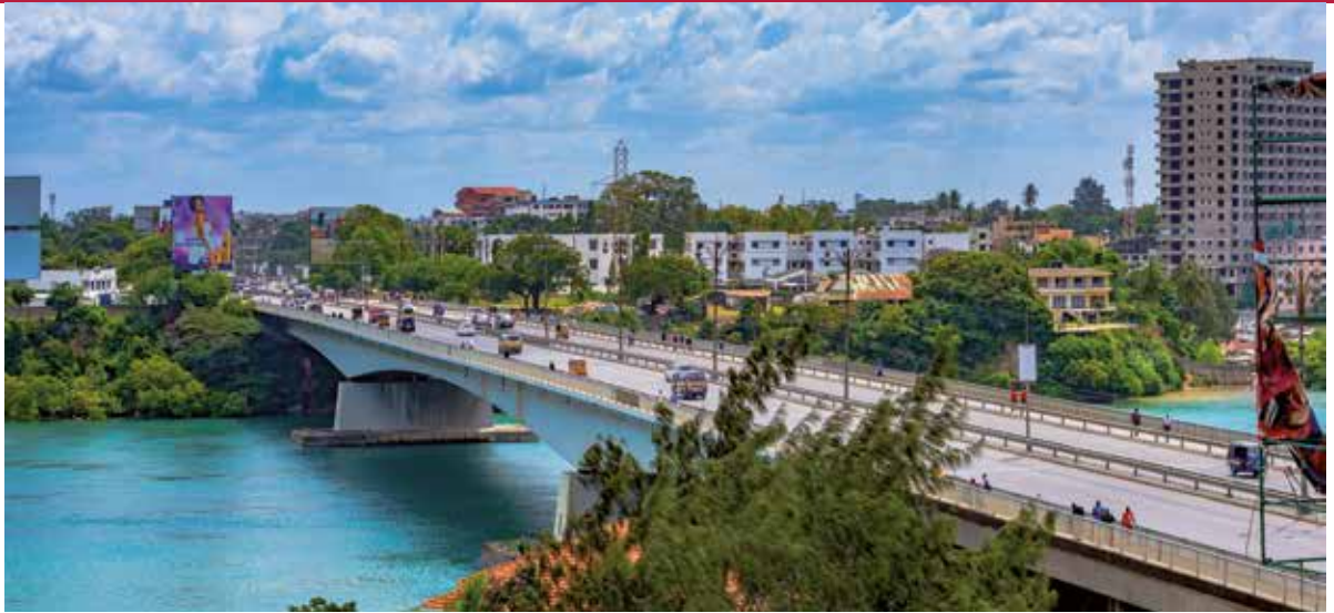
New Nyali Bridge in Mombasa, Kenya
